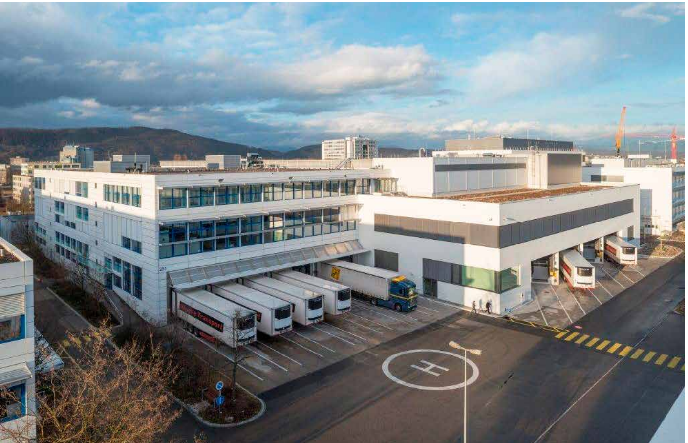
Exterior view of the warehouse and logistics centre of F. Hoffmann-La Roche Ltd in Kaiseraugst. The seven truck loading bays for normal-temperature materials are visible on the left, the four loading bays for chilled materials on the right.
